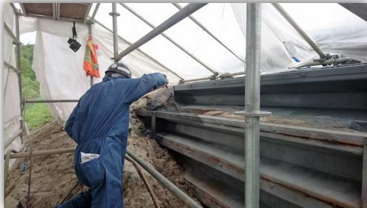
The refurbishing of a retaining wall on the Trans-Canadian highway completed in 2017.
